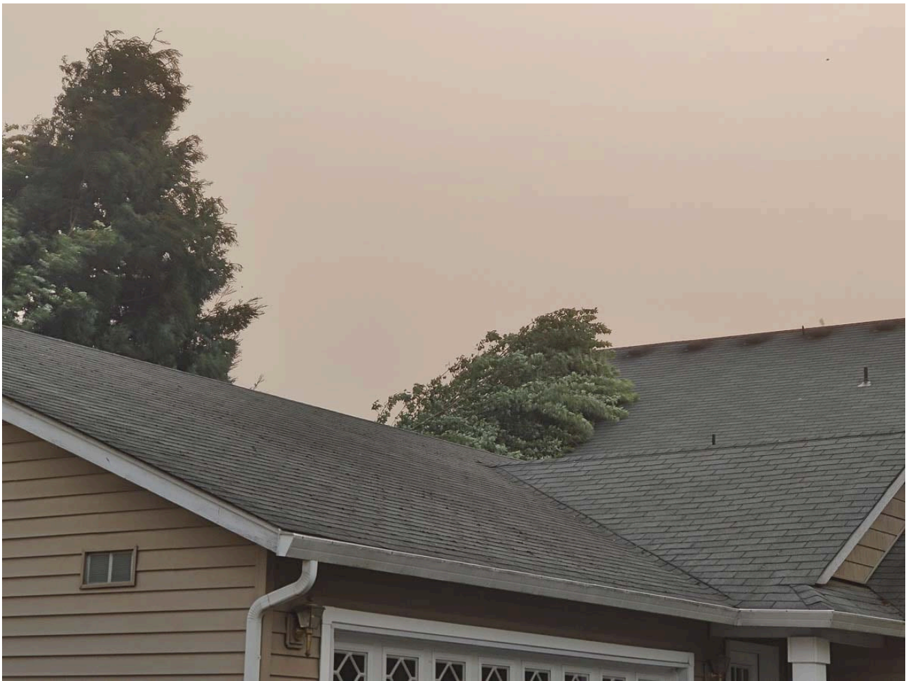
A tree rests against the side of a house in Battle Ground during a wind storm Monday evening. Photo by Chris Brown
